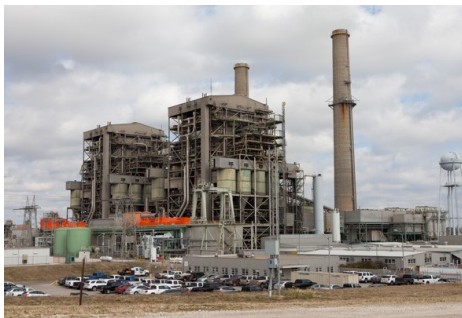
Big Brown power plant | Vistra Energy
