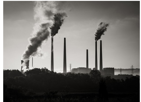
Sammis Power Plant | Robert S. Donovan / CC BY-NC 2.0
